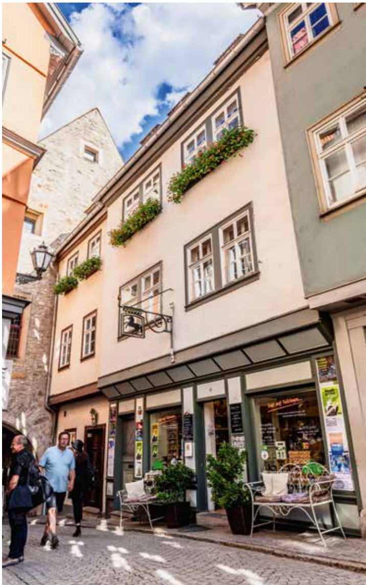
The Krämerbrücke (Merchants' Bridge) is Europe's oldest residential bridge. Already the Bachs took strolls here.
